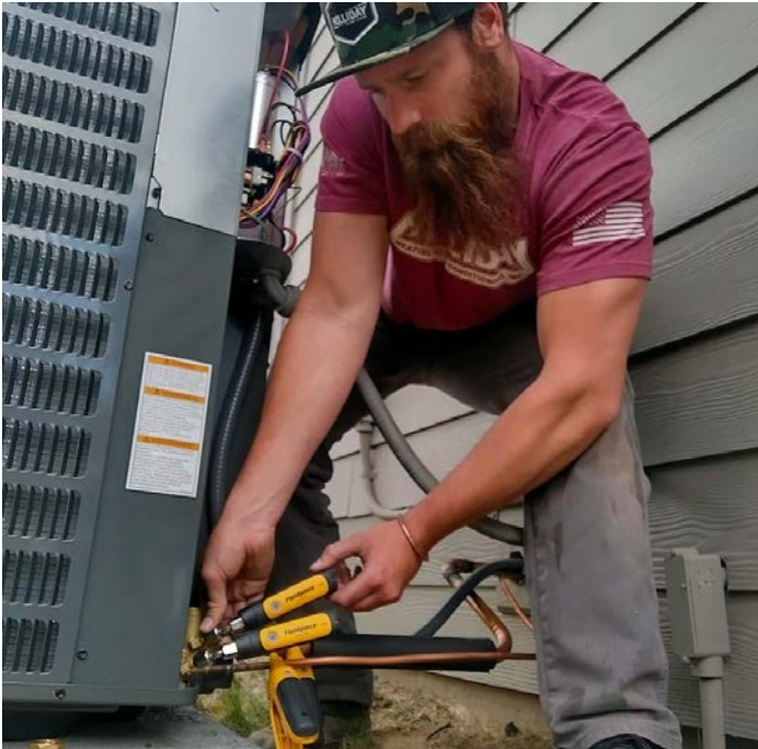
Figure 1. A Holliday technician secures a set of Fieldpiece JobLink probes to measure refrigerant pressure and temperature of an HVAC unit (Photo courtesy of Chris Holliday).
